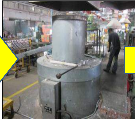
Electrical furnace with insulation 2013 – 14
