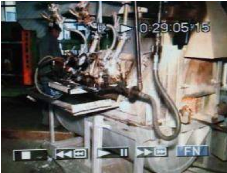
LDO Fired Baffco Furnace
