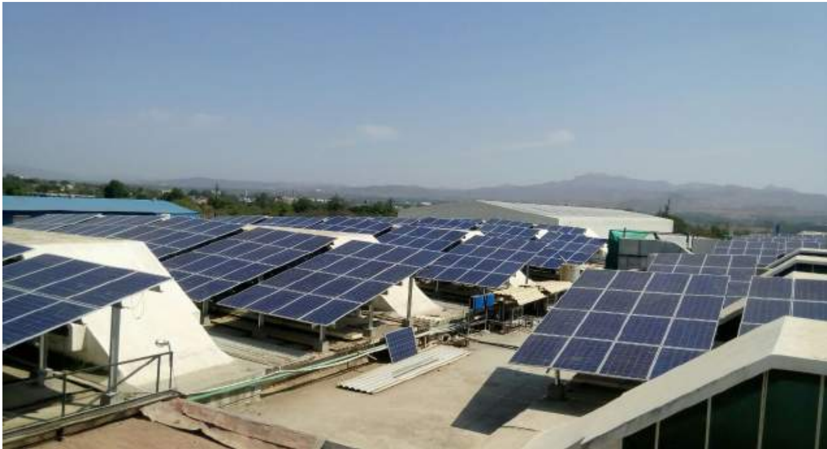
Solar Roof Top System- 250 KWp Capacity
